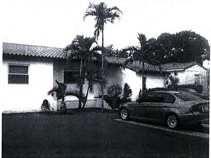
08-04-2014 HOUSE RIGHT SIDE VIEW
