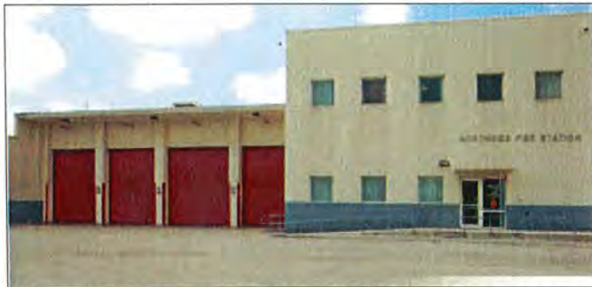
MIA Northside Fire-Rescue Station 59 serving the City of Miami Springs
