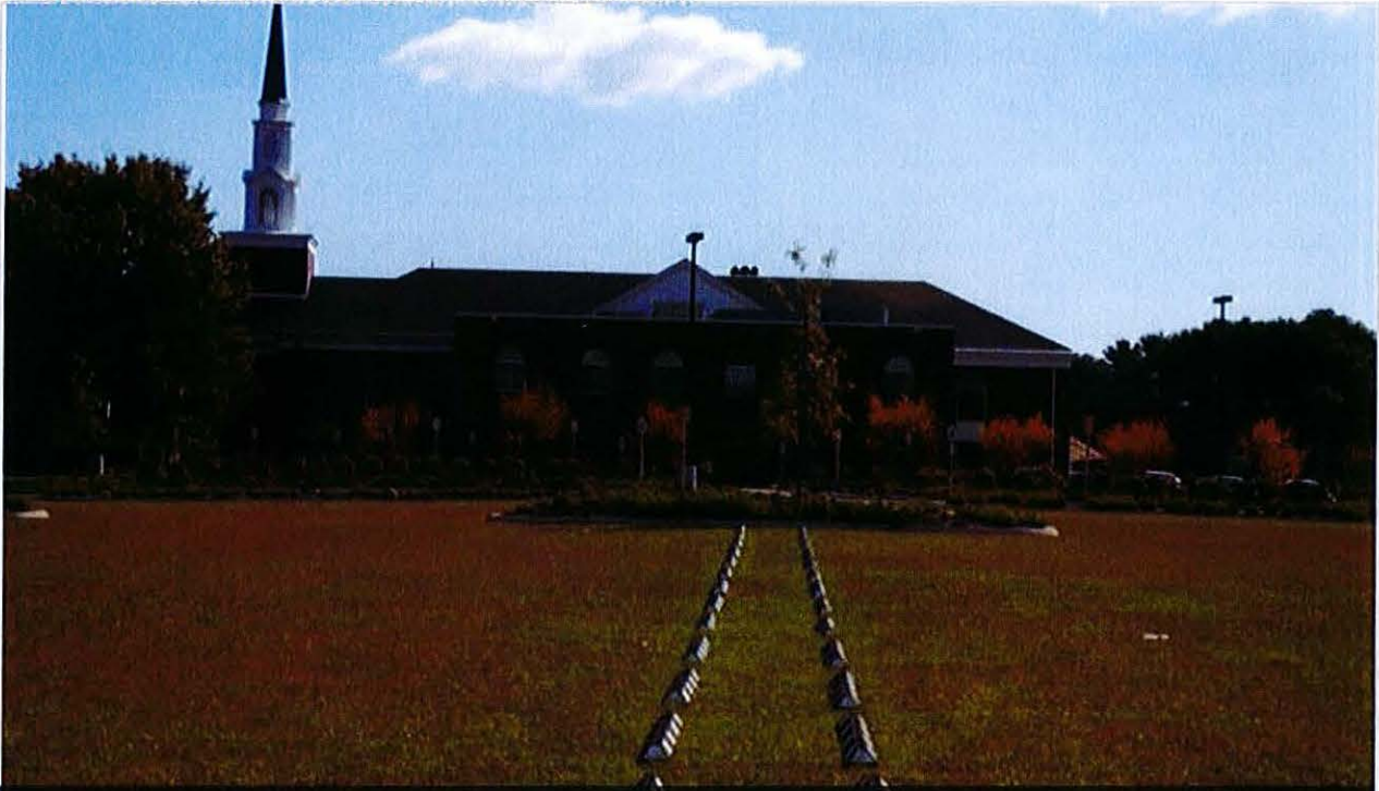
Completely vegetated Geoblock grass pavement system. Parking spaces delineated with markers.
