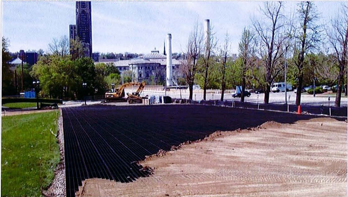
Installation of the Geoblock porous pavement system for a grassed overflow parking area.
