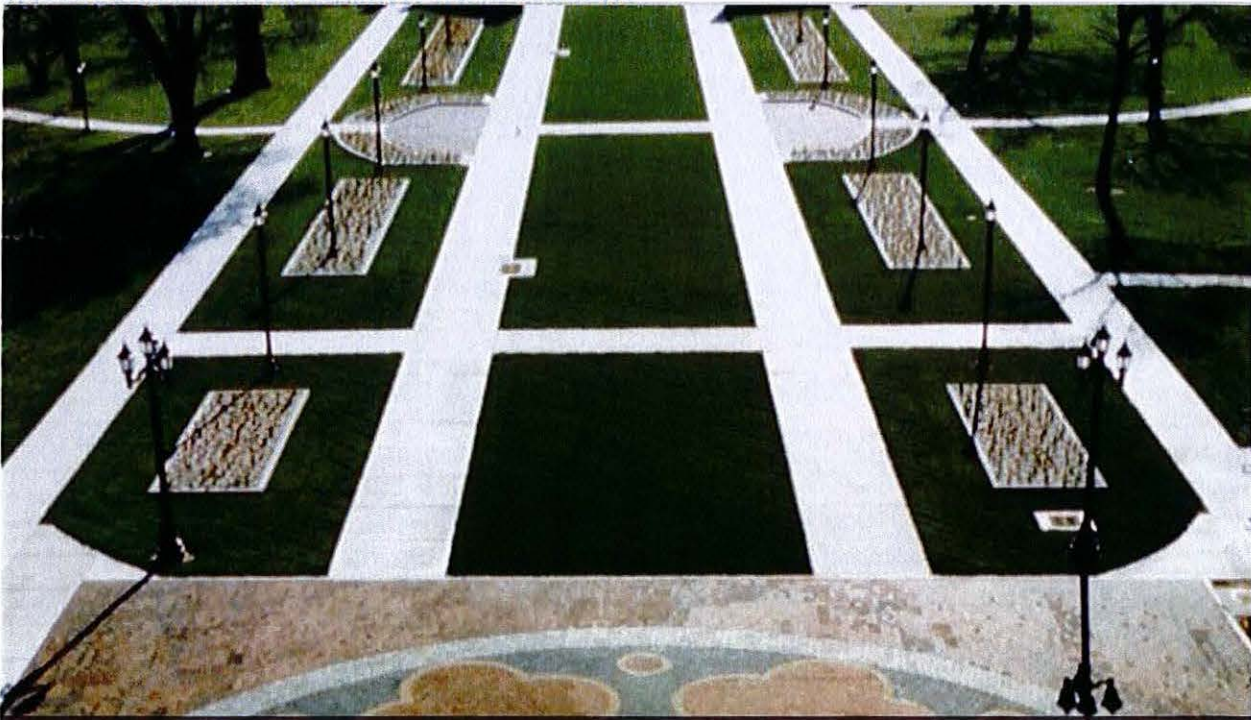
A grassed parking area at a university utilizes the Geoblock porous pavement system.
