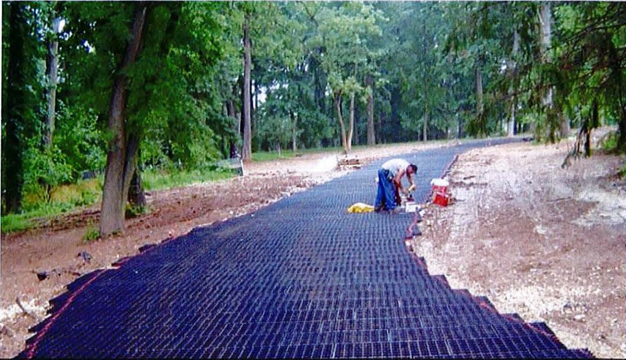
Placing the Geoblock system in a bricklayer pattern on a roadway curve.
