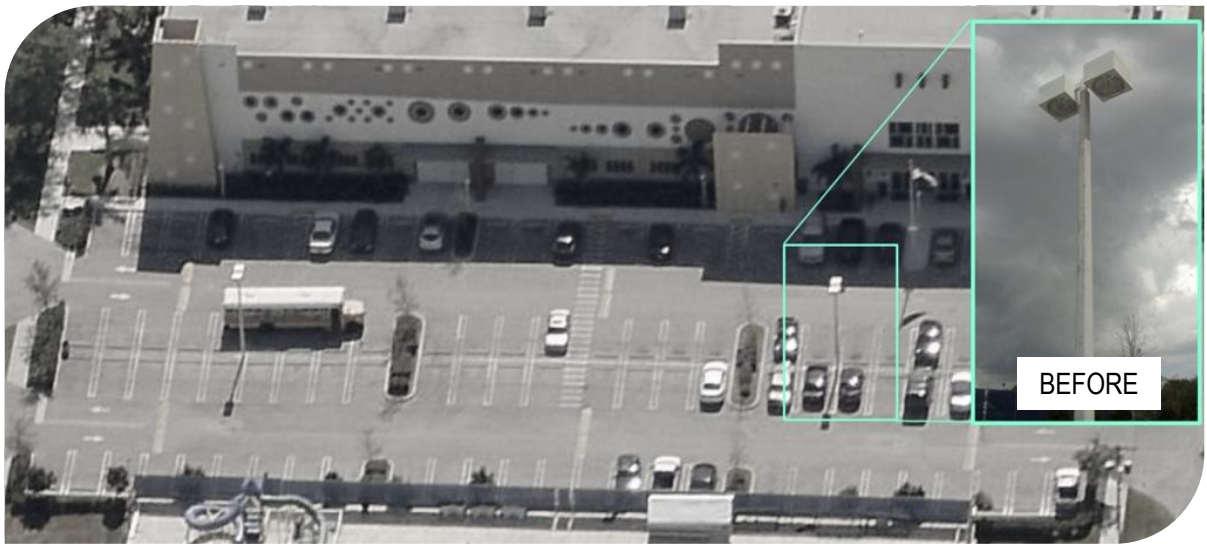
Miami Springs Community Center Parking Lot (Inset Photo - Existing HPS fixture installed on existing pole)
