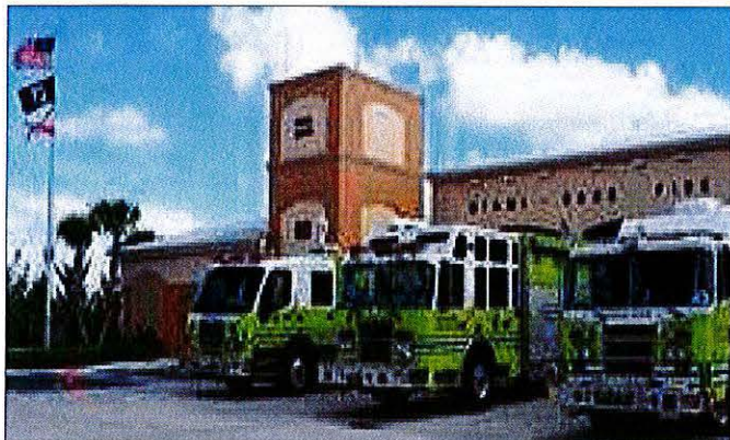
Doral North Fire-Rescue Station 69
