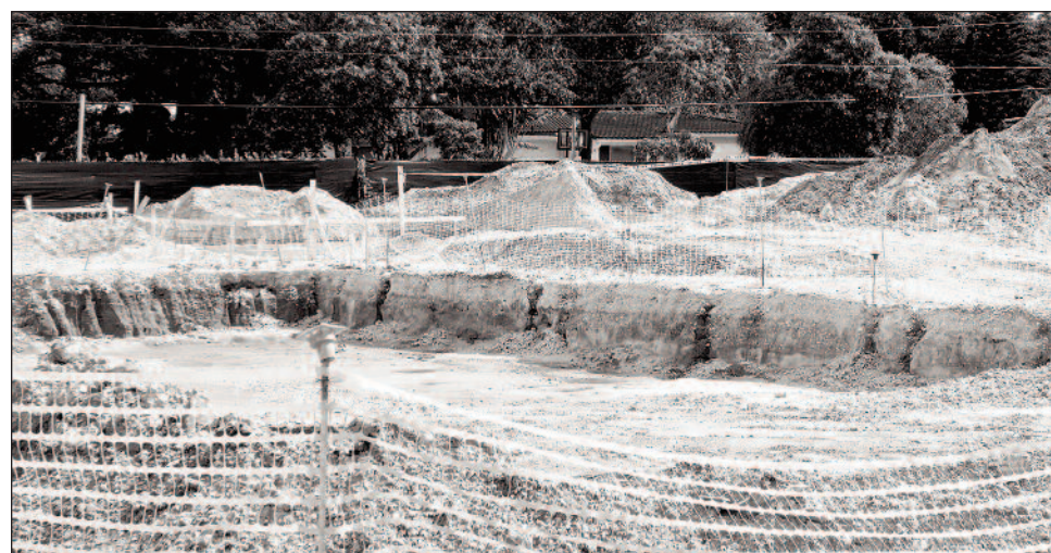
Excavation and foundation preparation are underway for the new Aquatic Center.
