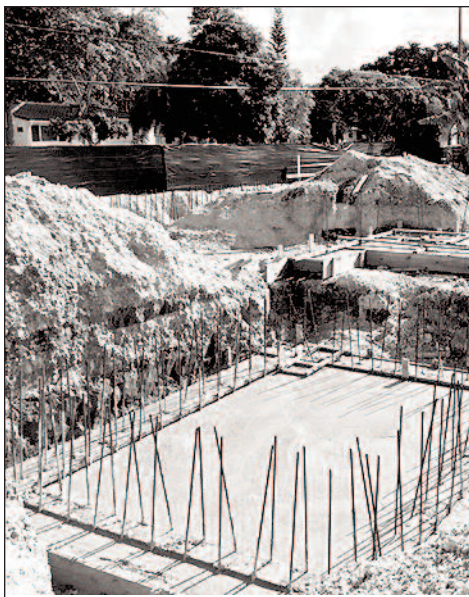
Restrooms and locker areas are taking shape.
