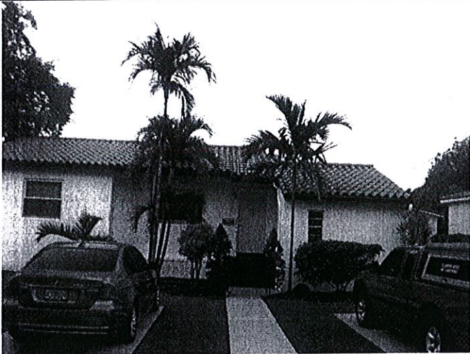
08-04-2014 HOUSE FRONT VIEW
