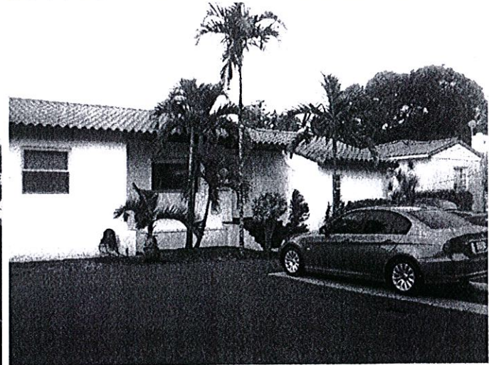
08-04-2014 HOUSE RIGHT SIDE VIEW
